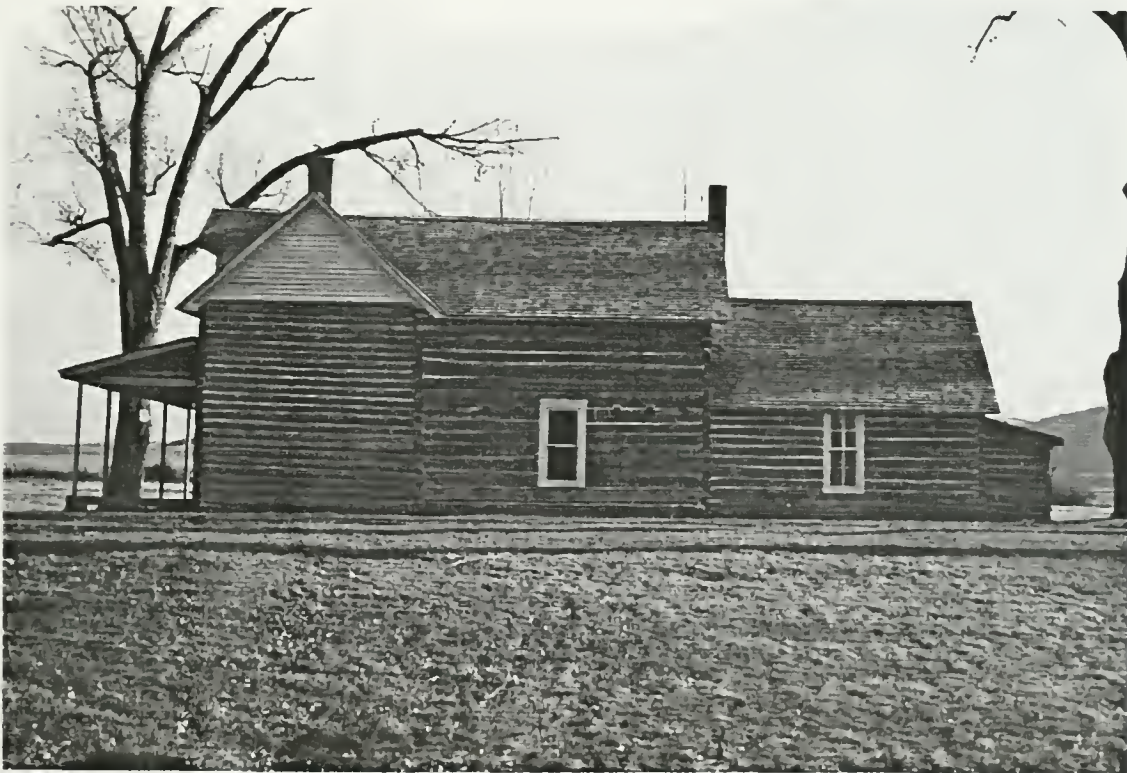
View of west facade of Chief's House.
